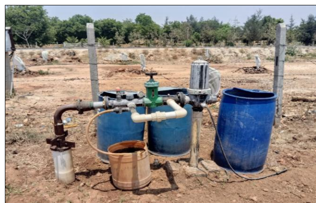
Fig 1: Venturi fertigation system setup in the experimental field plot
