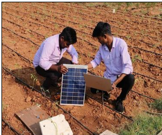
Plate 2: Installation of solar panel
