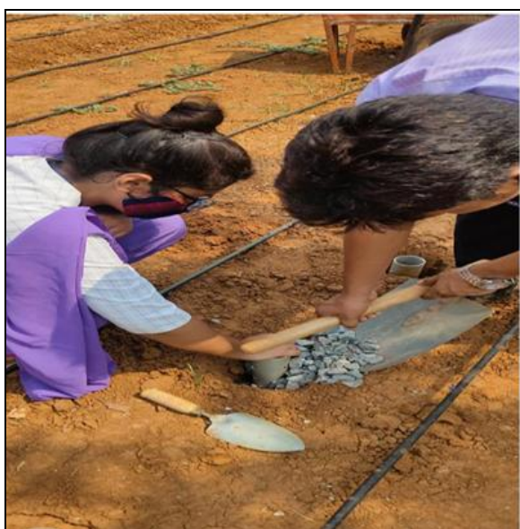
Fig 3: Filling the Gravels
