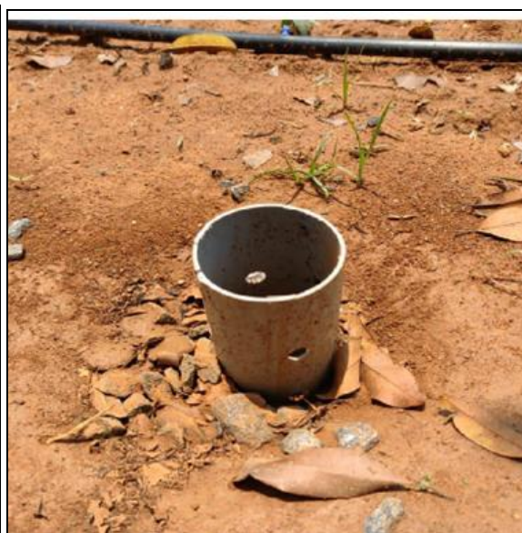
Fig 4: PVC Pipe Installed
