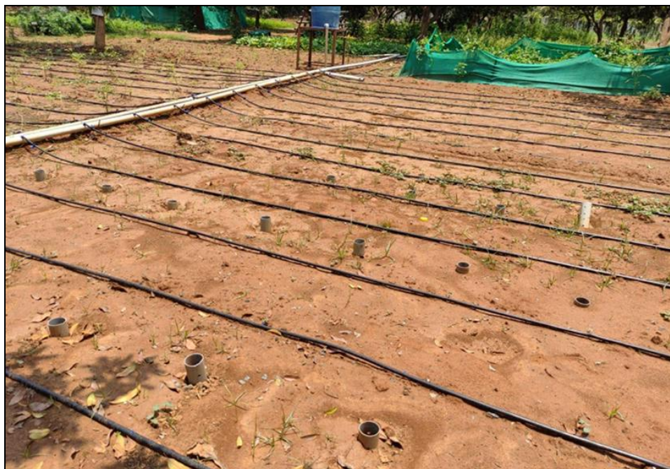
Fig 5: Installation of Drilled PVC Pipe (0.7 m depth)
