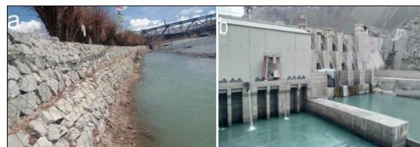
Fig 6: (a) Steel net stone cage river embankment on river Indus (b) Nimo- Basgo Hydro project at Basgo village.
