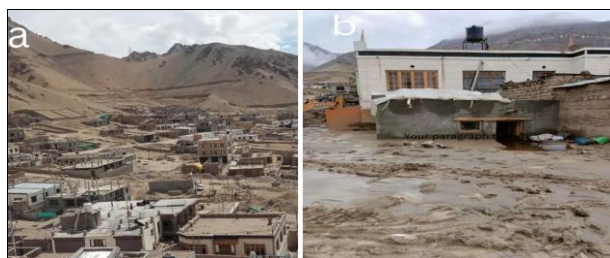
Fig 5: Houses constructed on the hill slopes the Skampari area in Leh city (b) Debris flow damage houses in skampari in august 2024 cloudburst.
