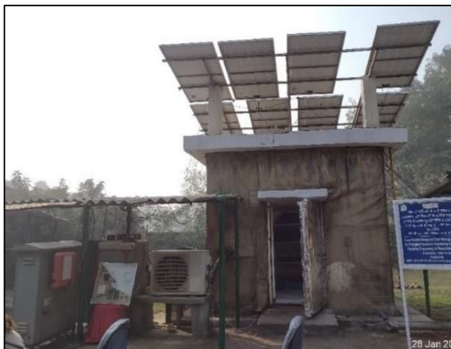
Fig 1: A view of the SREC structure
