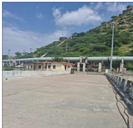
Fig 3: Bisalpur Pipe line
