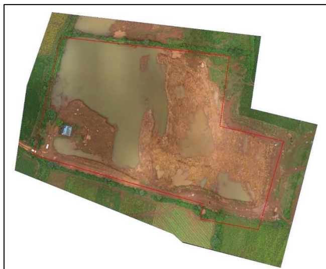
Fig 1: Orthomosaic image obtained from drone processing, displaying the excavated portion of the mining lease and the water-filled areas.
